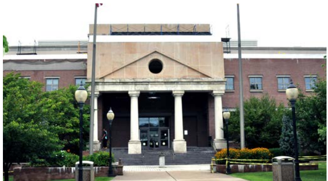
The Hunterdon County Justice Center in Flemington as it appears today.
